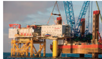
Fields of promise: The nine deep offshore sites (left); the Horns Rev 2 accommodation platform is lowered into place (right)
